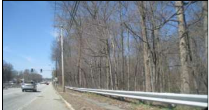
Guardrail located on the ‘private’ side of the sidewalk.
