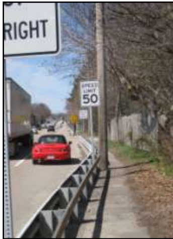
Guardrail located between Route 9 and sidewalk.
