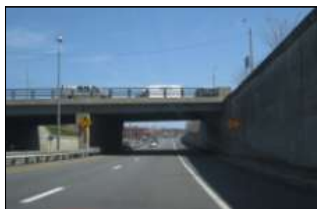
Overpasses along Route 9 in Wellesley
