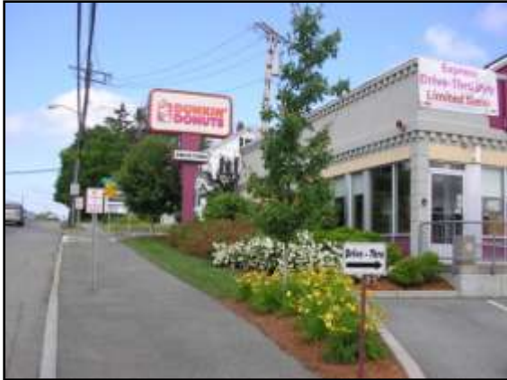
Retail business in Framingham with building sited near Route 9 and a well-landscaped buffer. Parking is at rear of building.
