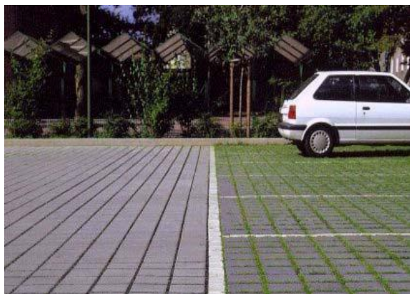
Parking reserve with permeable pavers
