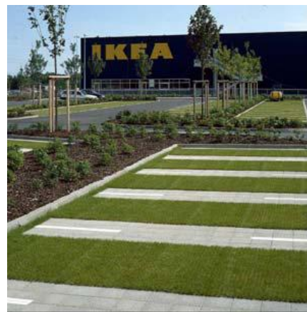
Parking lot with pavers and grass
