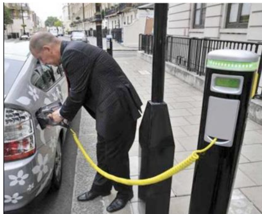
Another style of electric charging station
