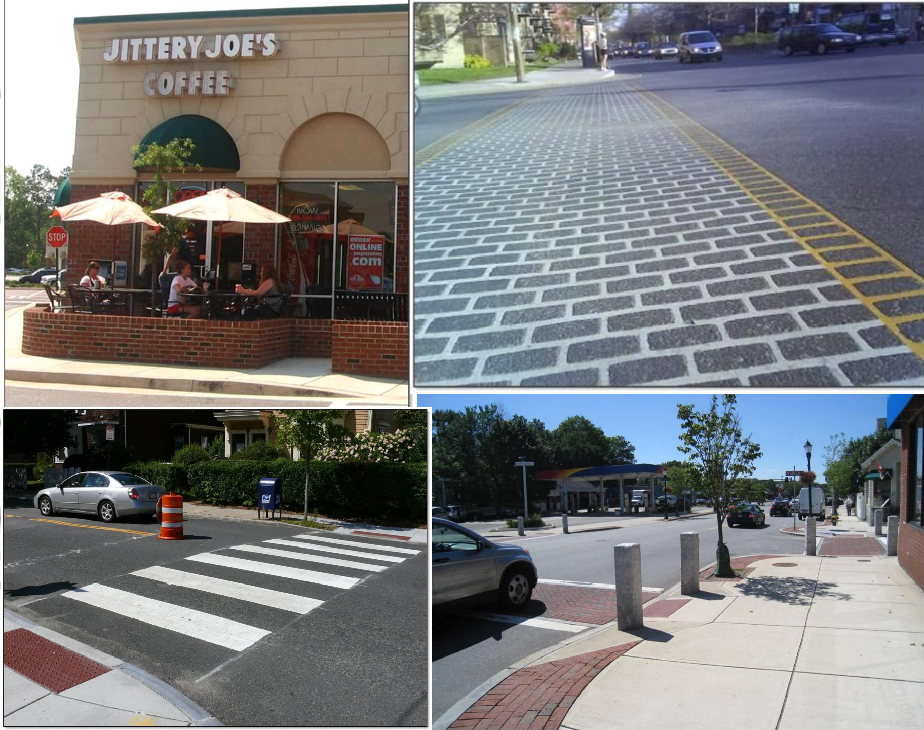
Crosswalks with bumpouts, outdoor seating, wide sidewalks
