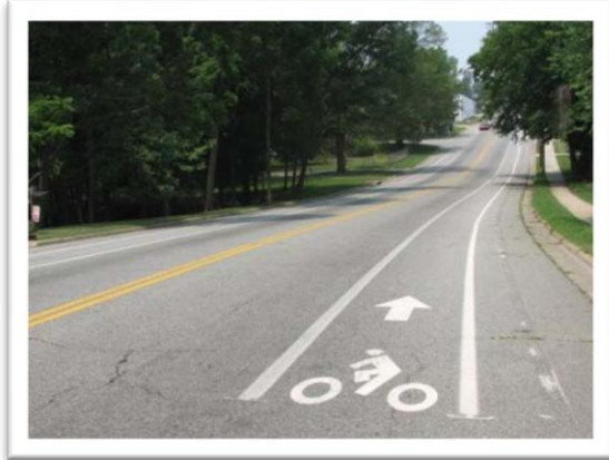
Figure 23 Example of a Bicycle Lane
