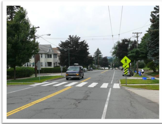
Figure 28 Curb Extension – Image and Graphic
