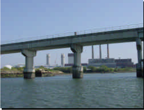
MBTA Commuter Rail Bridge
