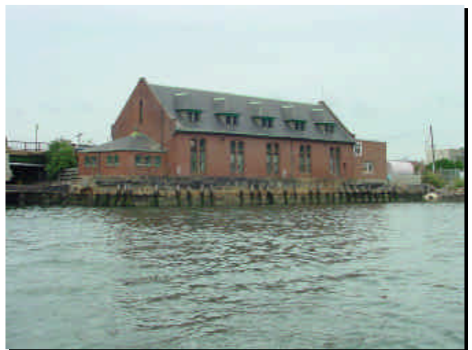
Boston Water and Sewer Commission Pump Station
