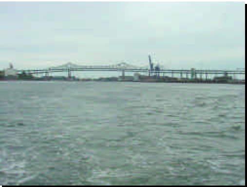
Tobin Bridge looking south
