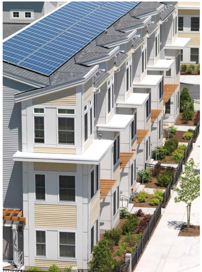
Solar panels on Old Colony BHA housing
