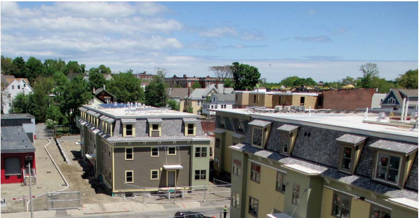
This Choice Neighborhoods development includes a six unit, new, net-zero energy use building on Quincy Street, Roxbury. All buildings will qualify for LEED Silver or higher energy rating.
