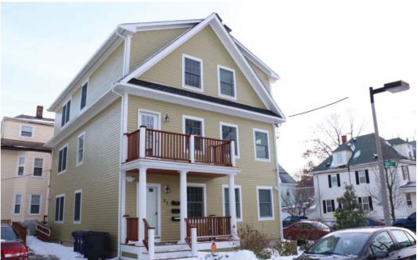
81 Brent St: This LEED Platinum home in Dorchester is 45% more energy efficient than the average home.
