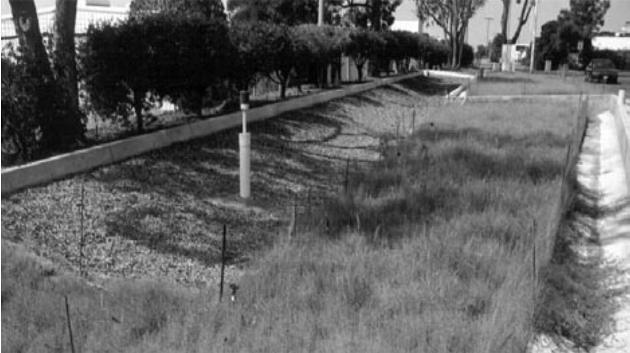
Above: Here a filter strip is being used as pretreatment for parking lot runoff directed to an infiltration basin. Note concrete level spreader (at right) to facilitate sheetflow across filter strip. *Photo: California Stormwater Quality Association*
