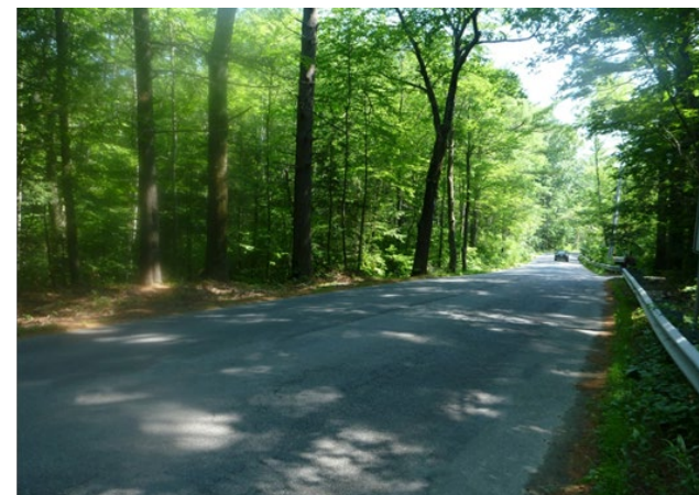
Example of a road with no centerline or other striping
