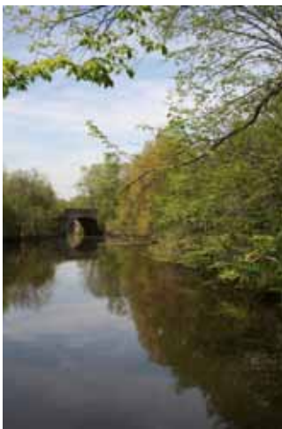
View of the Boston Avenue Bridge
