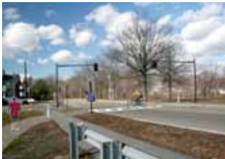
Access improvements at (from top) West Medford MBTA commuter rail stop, Boston Avenue, Boston Avenue East, and Decatur Street
