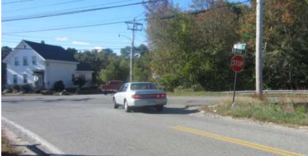
Vehicles on Cross Street stop at Main Street edge line (well beyond stop sign) for improved visibility
