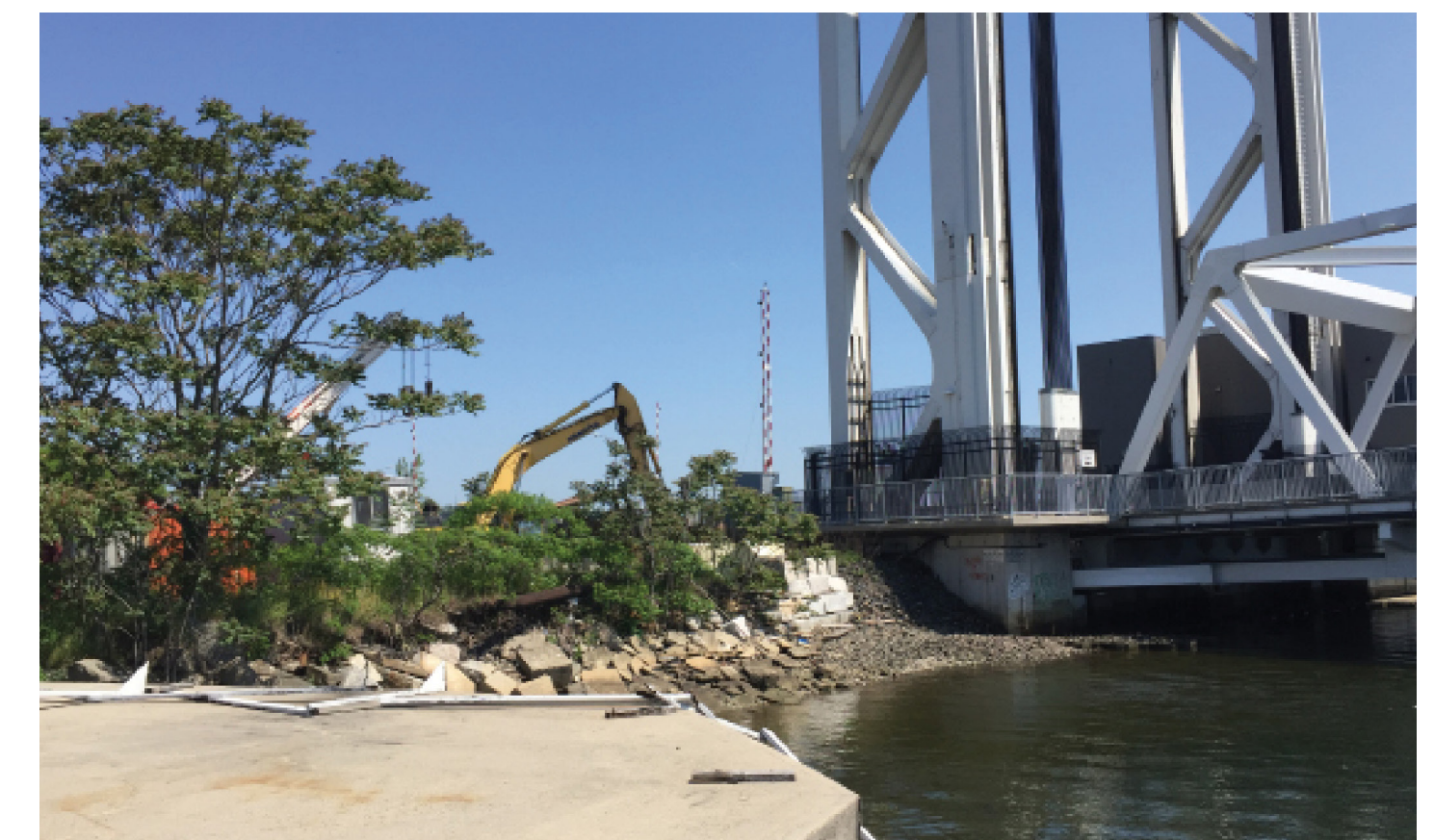
Parcel south of Chelsea St Bridge (looking north)
