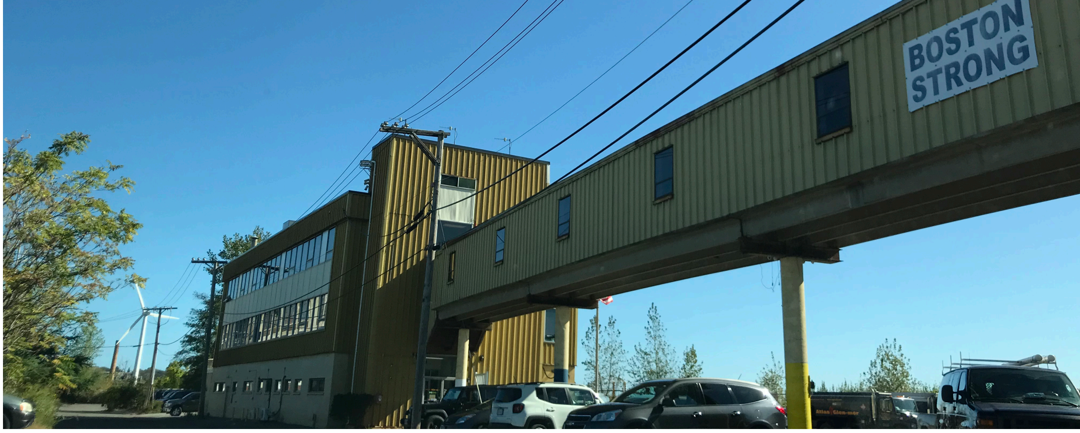
Eastern Ave Extension site
