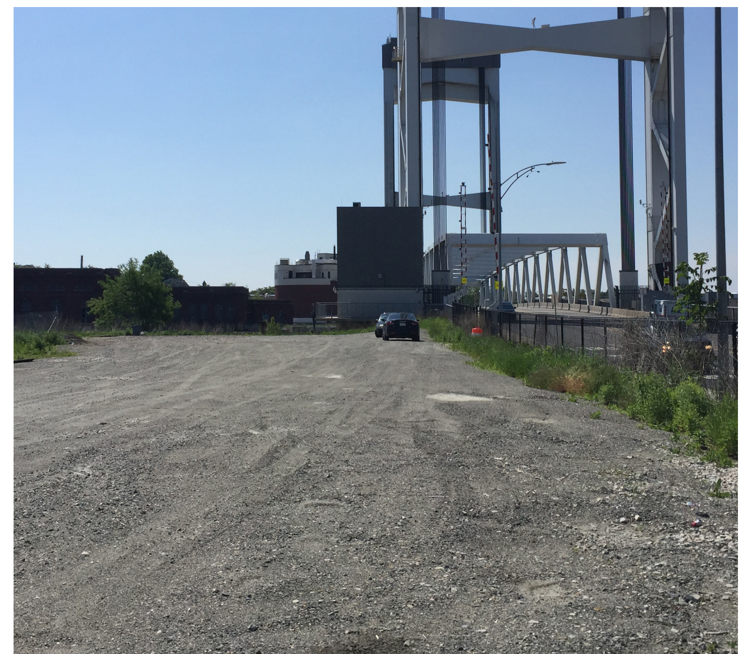
5. Underutilized land at next to the Chelsea St. Bridge
