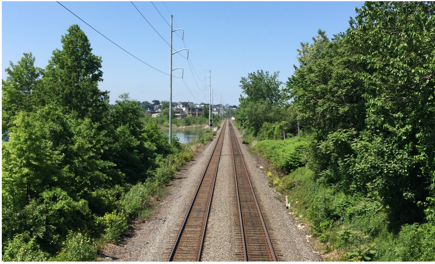
Commuter Rail tracks
