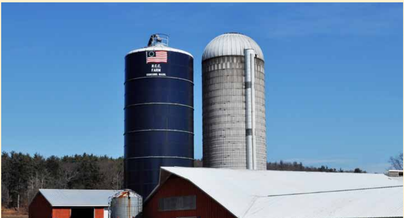
The barn and silos at the Northeastern Correctional Center’s Prison Farm. Much of the newer infrastructure was built by Dave and inmates in the 1980s.
