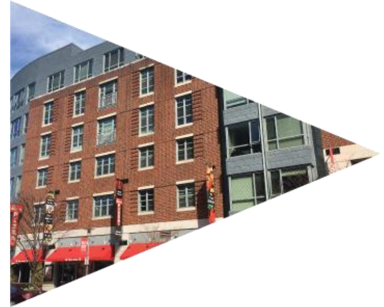
Additional Housing Demographics
