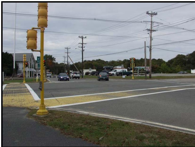
This is a busy intersection that experiences some delays, primarily due to the lack of designated left-turn lanes and left-turn signal phases. The widths of the approaches on Route 140 do not accommodate turning lanes. Motorists on the Route 140 southbound approach to Route 1A can bypass the intersection by using Bank Street as a slip lane.
