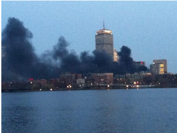
Back Bay, Boston, substation fire, 2012
