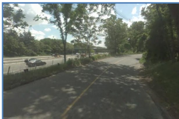
Figure 16 Route 128 in Weston
