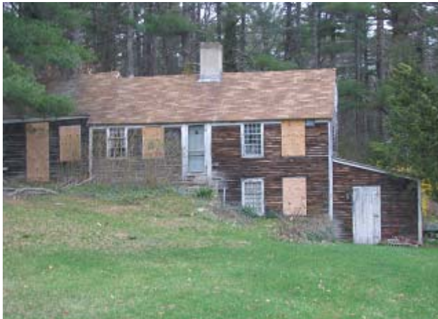
Boarded-up house, Plympton
