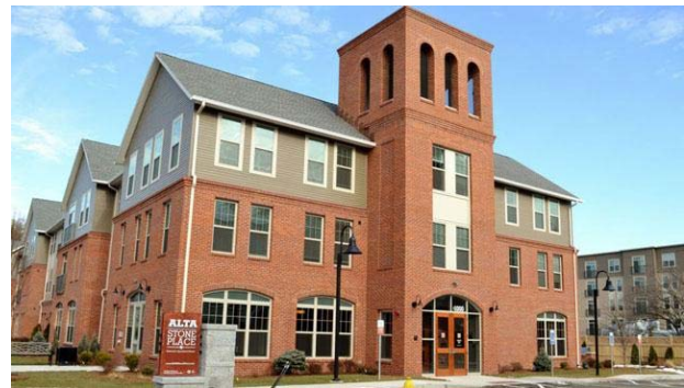
Figure III-4 – Alta Stone Place
