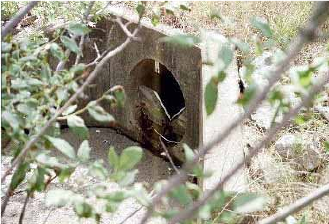
Figure 4-1 Route 9 Stormwater Outfall to South Pond
