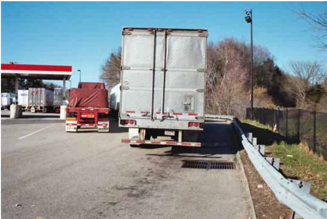
Figure 4-7 Truck Stop in proximity to Catch Basin, Natick Service Plaza
