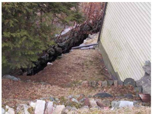
Note the downspout and the white drainage pipe draining directly to the stream
