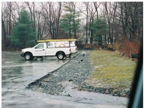
Drainage system is failing after winter ice & snow lifted the drainage pipes
