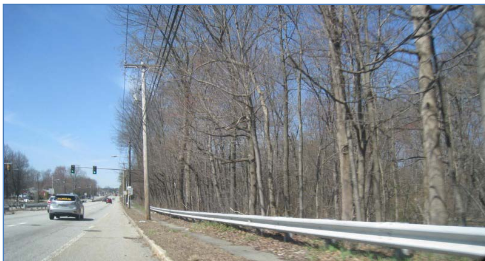
Examples of guardrail placement on the 'private side' of the sidewalk.
