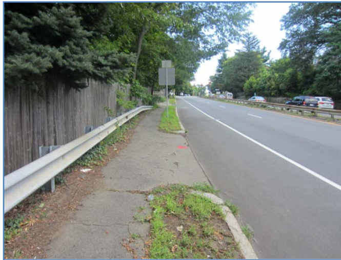
Example of a curb cut not providing access to a driveway or a street north side of Route 9 west of Oakland Street.
