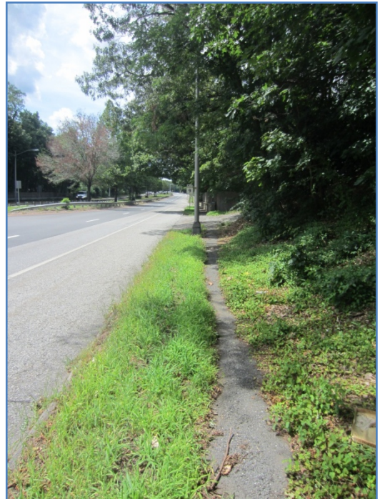
Examples of narrow sidewalks with significant vegetative overgrowth east of Cedar Street (left) and east of Audubon Road (right) on Route 9 westbound.
