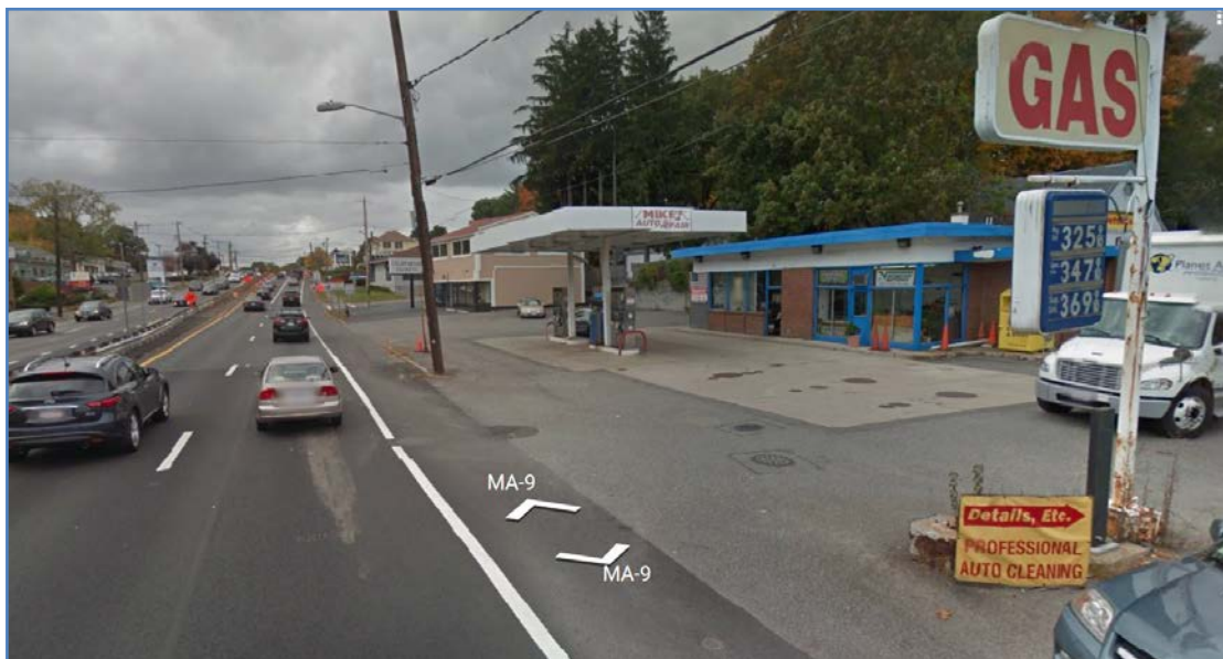
Example of a curb cut not providing access to a driveway or a street north side of Route 9 west of Oakland Street.
