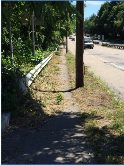
Examples of narrow sidewalks with significant vegetative overgrowth east of Cedar Street (left) and east of Audubon Road (right) on Route 9 westbound.
