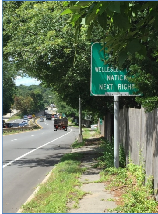
A common occurrence is signage obscured by vegetation, Such as this sign located near the Route 16 intersection.
