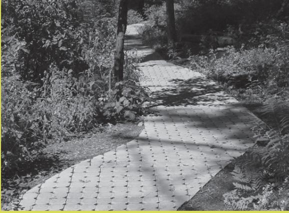
Above: A handicap-accessible park pathway made of permeable paving stones.
