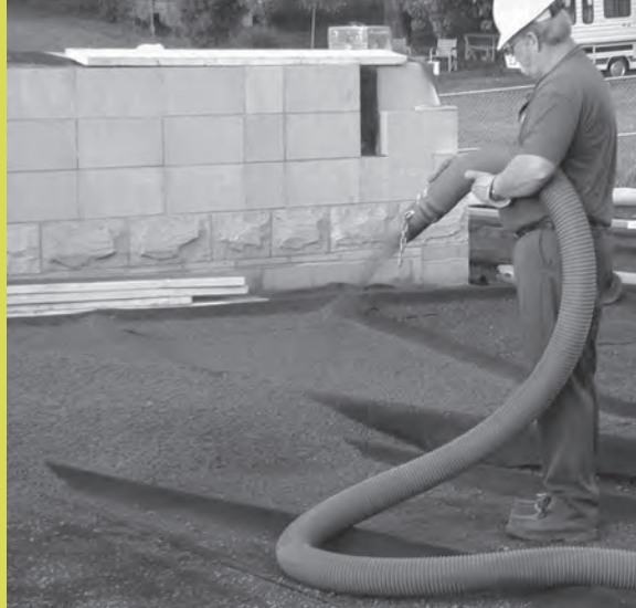
Above: Installation of eight inches of soil medium using pneumatic equipment at the Oaklyn Branch Library in Evansville, IN. Photo: © 2005, Roofscapes, Inc. Used by permission; all rights reserved.
