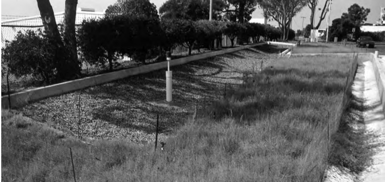
Above, and Cover: The parking lot runoff directed to this infiltration basin is pretreated by a vegetated filter strip. Note concrete level spreader (at right) to facilitate sheetflow across filter strip. Photo: California Stormwater Quality Association
