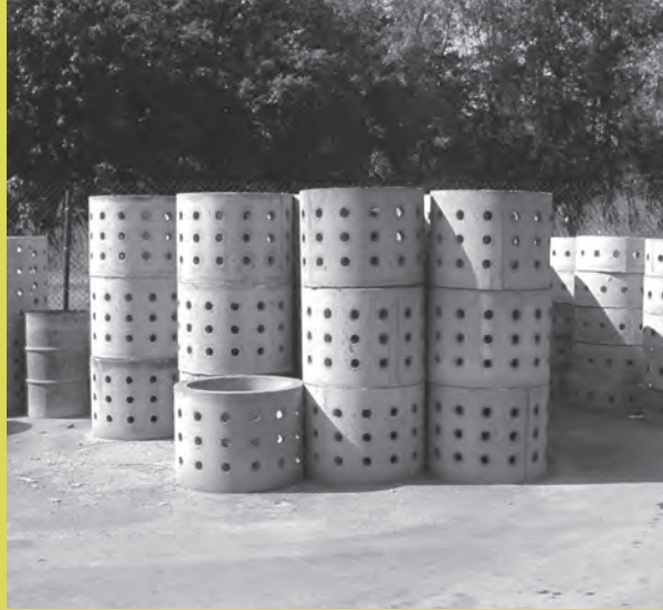
Above: Precast concrete drywell inserts prior to installation. Photo: Lower Columbia River Estuary Partnership
