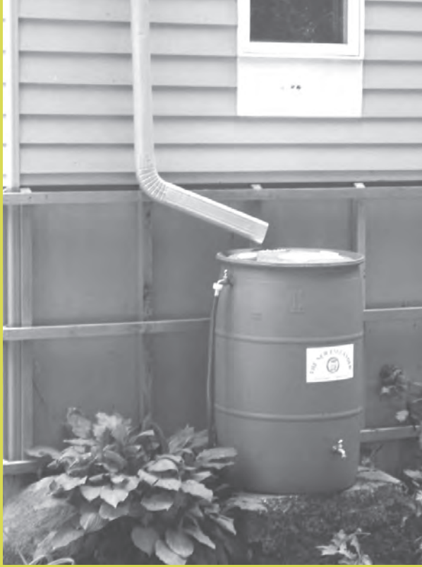
The overflow outlet from this rain barrel drains into an adjacent rain garden. Photo: GeoSyntec Consultants, Inc.
