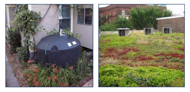
These on-site management features can address stormwater quantity and quality, and begin to reduce demands for municipal stormwater management. More information about these and other techniques, including the integration of recharge into an entire site's design, can be found in MAPC's Low Impact Development Toolkit.
