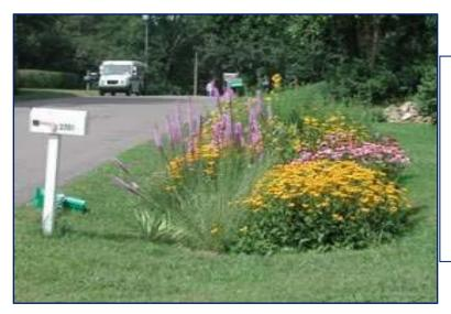
Raingardens slightly differ from Bioretention facilities because they typically do not involve amended soils, complex sizing calculations, or sophisticated conveyance devices (flow splitters, underdrains, overflow inlets, etc.) Rather, they usually a shallow depression in native soils, or modestly amended soils.
