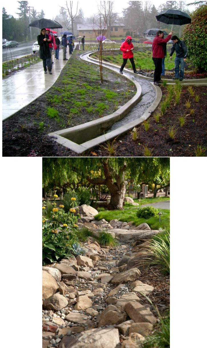
Figure 23 “Dry” beds or stream beds that manage stormwater as art installations.
