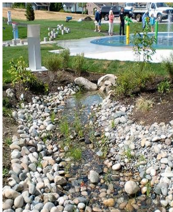
Figure 22 Created wetland that stores, cleans, and infiltrates spray feature wastewater.
