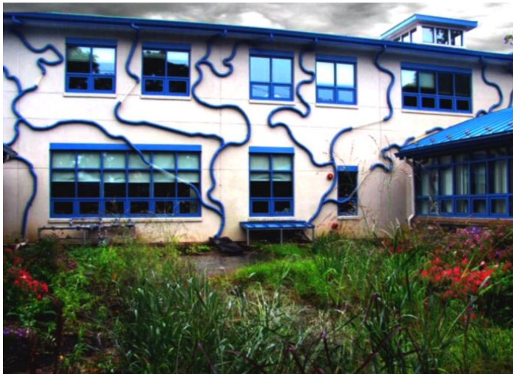
Figure 24 Rain water capture with artistic gutters and rain gardens.
