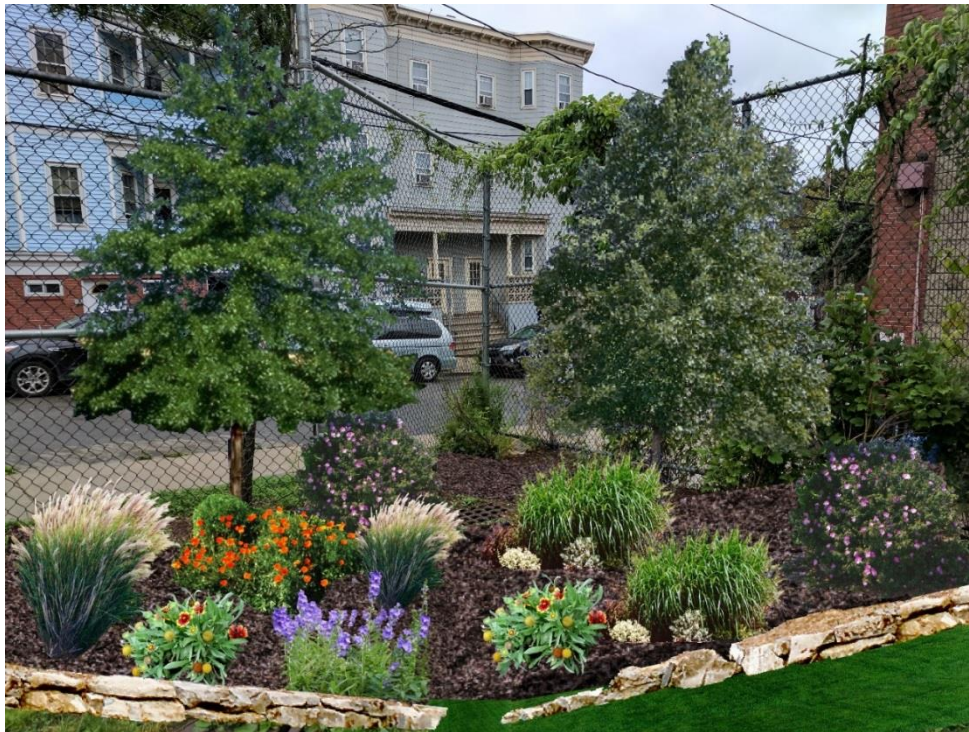
Figure 34 Quigley Park Bioswales and/or raingardens installed upslope of the storm drains but downslope of the park.
