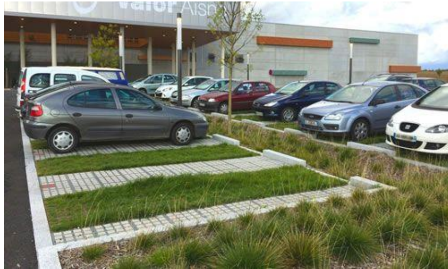
Figure 20 Green Parking Lots that capture stormwater and promote evapotranspiration for cooling the urban heat island.
