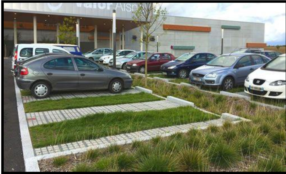
Figure 27 Green Parking Lots that capture stormwater and promote evapotranspiration for cooling the urban heat island.
