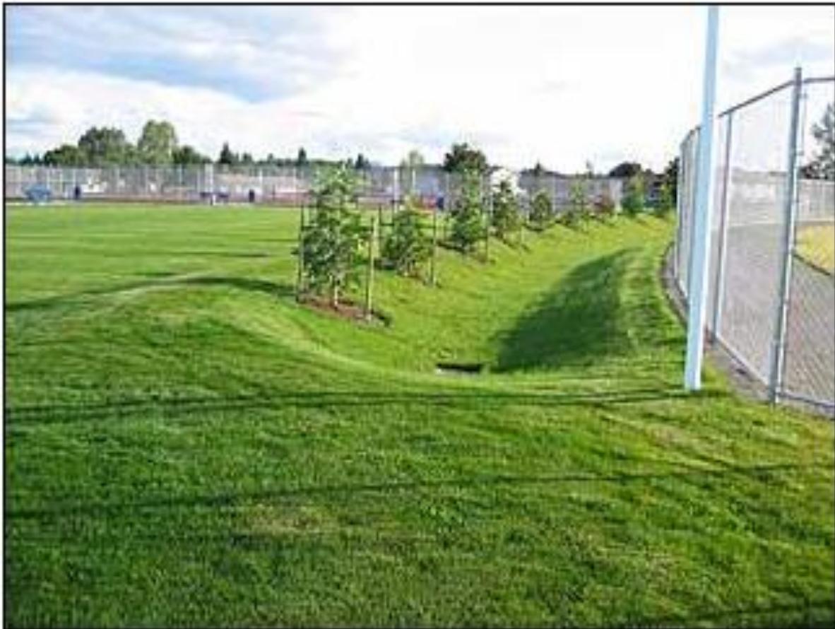
Figure 32 Example of natural stormwater infiltration infrastructure between playing fields with tree planting.
