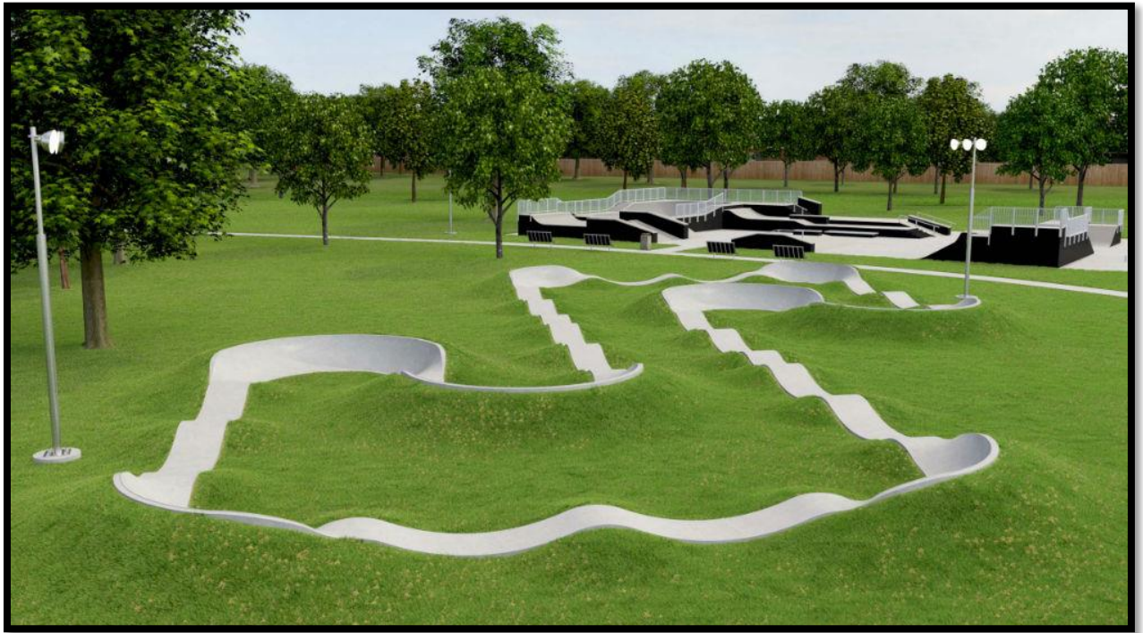
Figure 11 A pump track if designed correctly can serve as a recreation amenity and as flood storage infrastructure.
