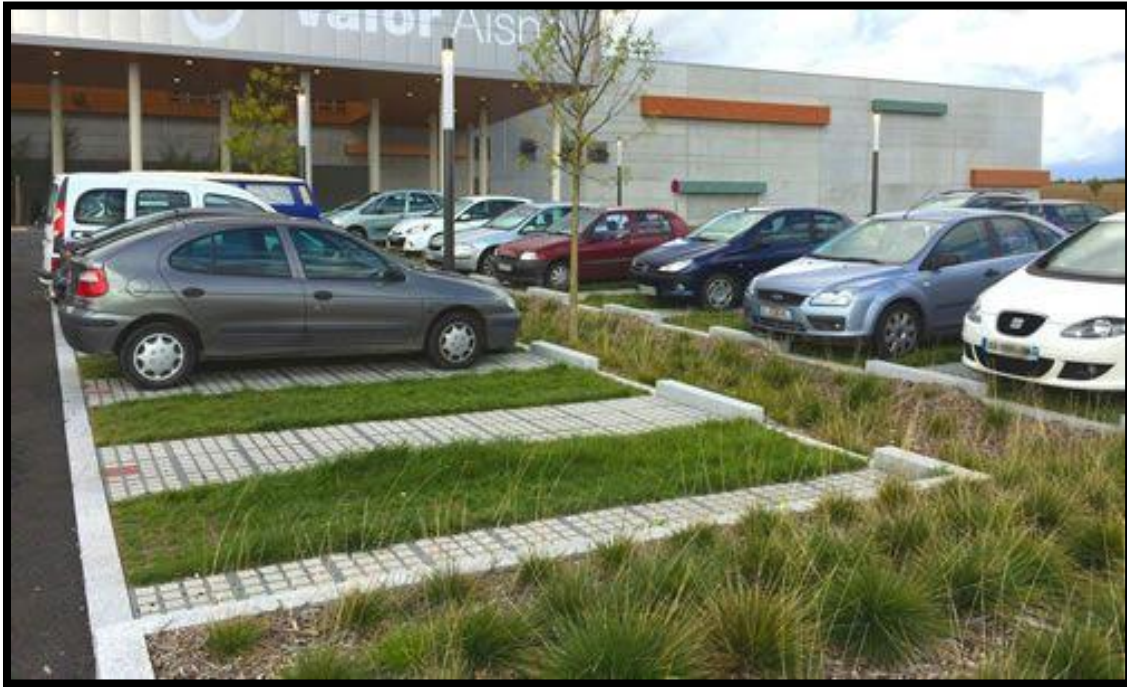
Figure 40 Green Parking Lots that capture stormwater and promote evapotranspiration for cooling the urban heat island.
