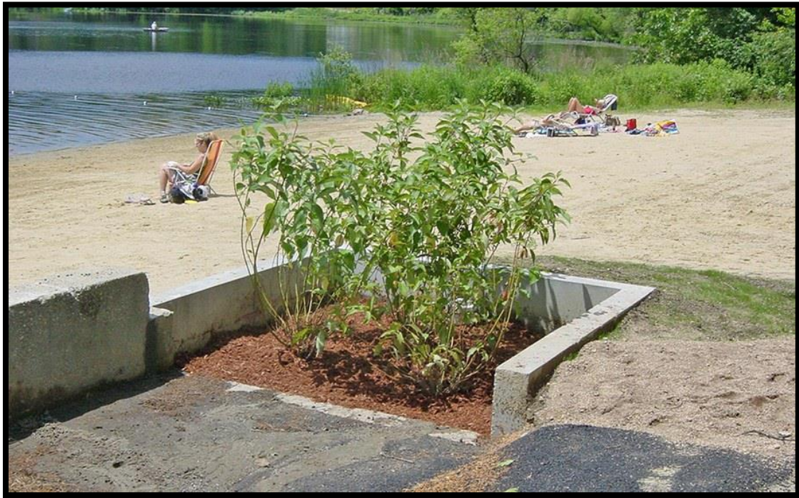
Figure 45 Stormwater directed to bio-retention basin, Long Pond, Littleton, MA.
