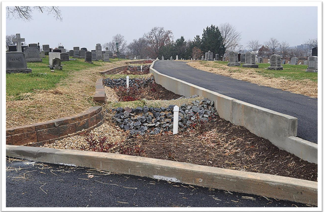
Figure 33 Bio-retention area installed at a narrowed drive at Mount Olive Cemetery, Washington, DC.
