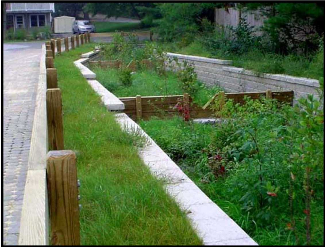
Figure 44 Vegetated swale with erosion control walls, Long Pond, Littleton, MA.
