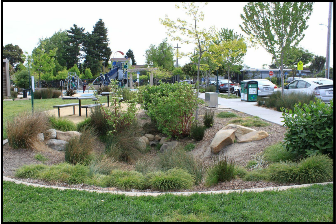
Figure 34 Bio-retention integrated into Doyle Hollis Park, Emeryville, CA.
