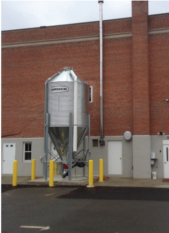
Pellet storage hopper installed at Northfield Town Hall
