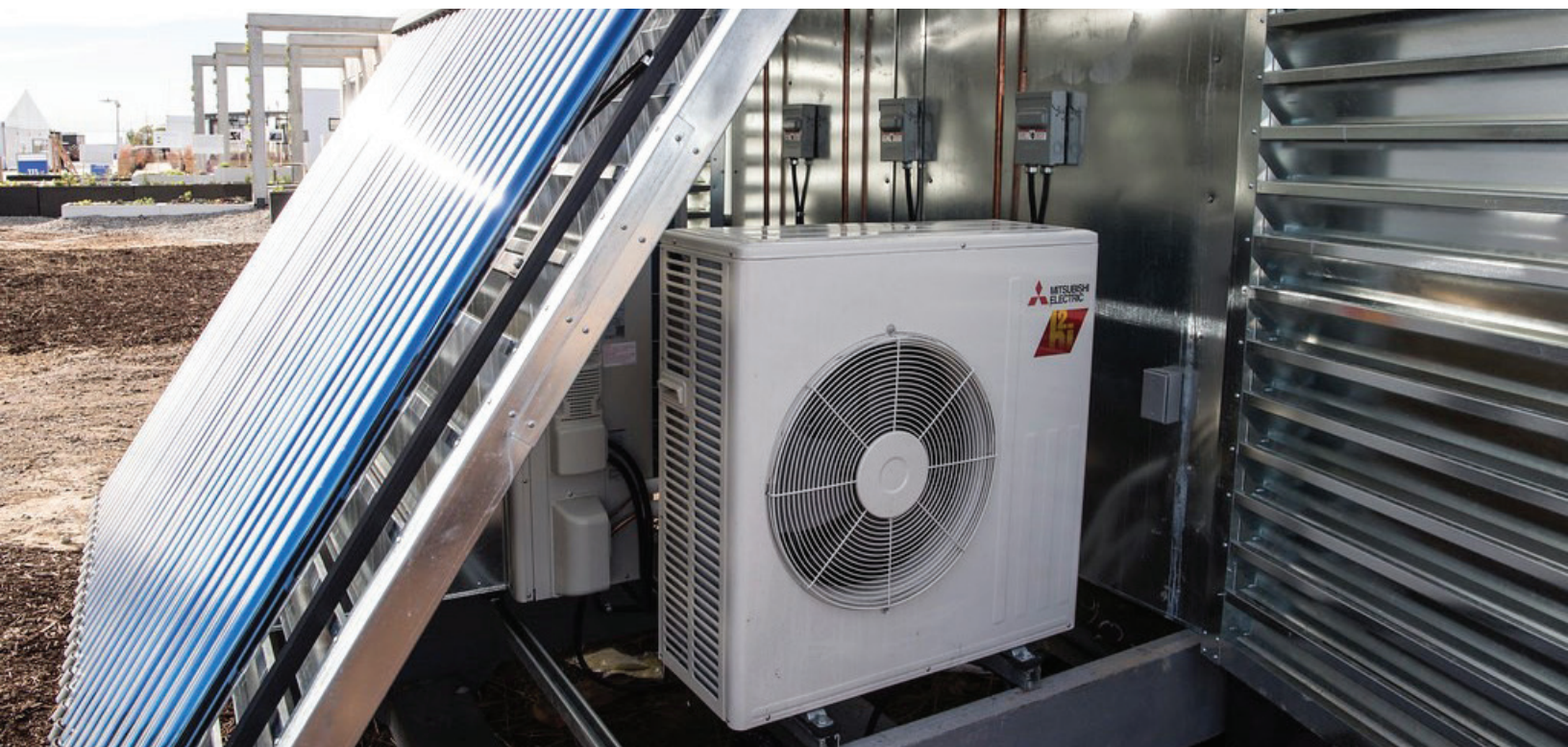
Solar thermal and an air-source heat pump. Source: National Renewable Energy Lab.
