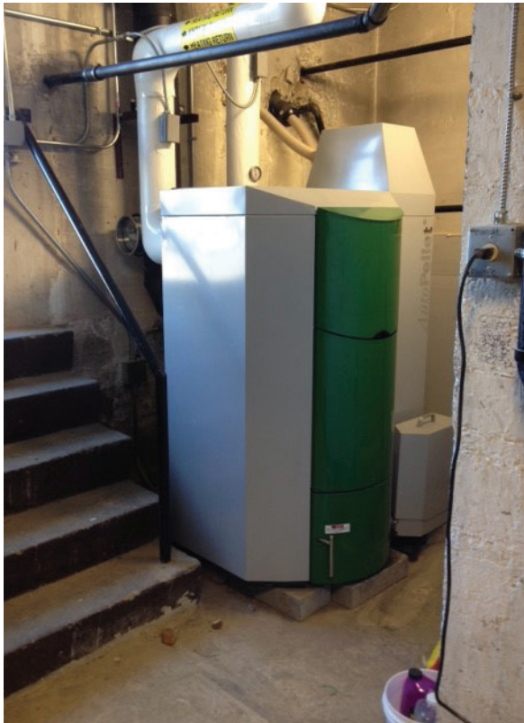
Pellet boiler installed at Northfield Town Hall
