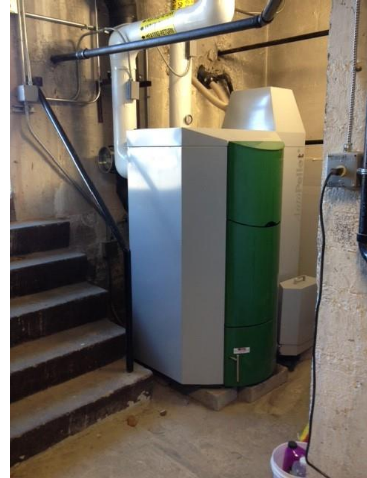
Pellet boiler system at Northfield Town Hall. Credit: Town of Northfield.
