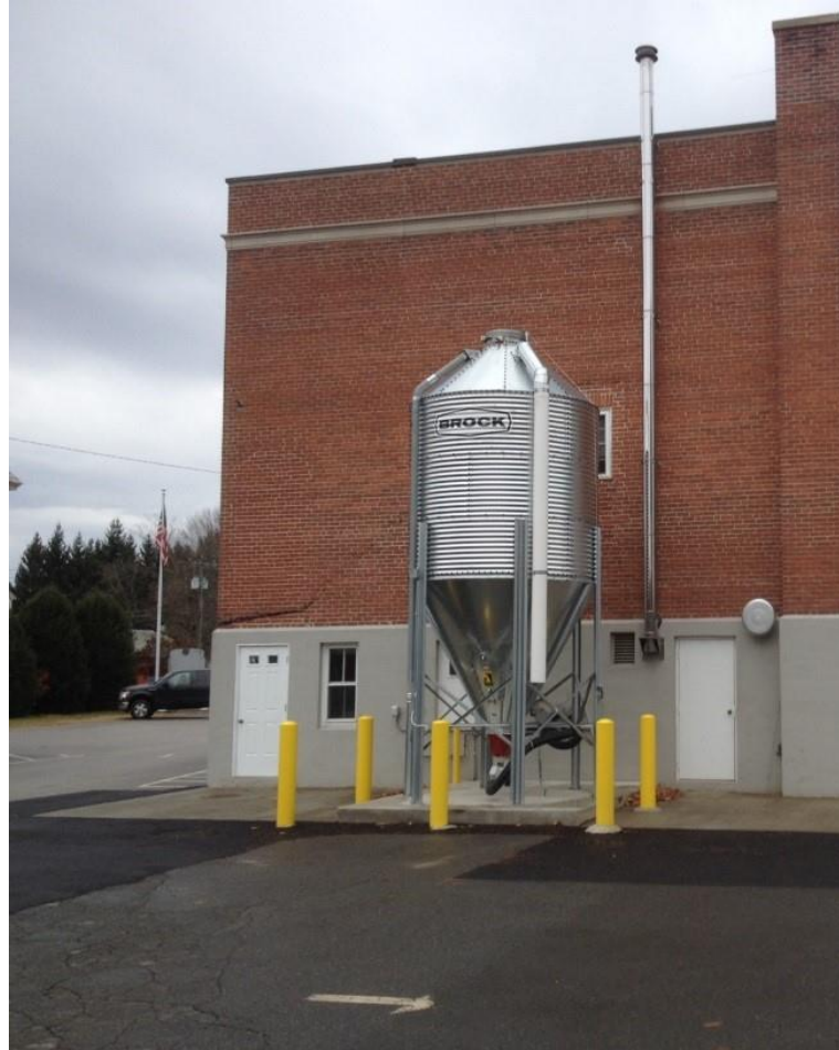
Pellet boiler system at Northfield Town Hall. Credit: Town of Northfield.
