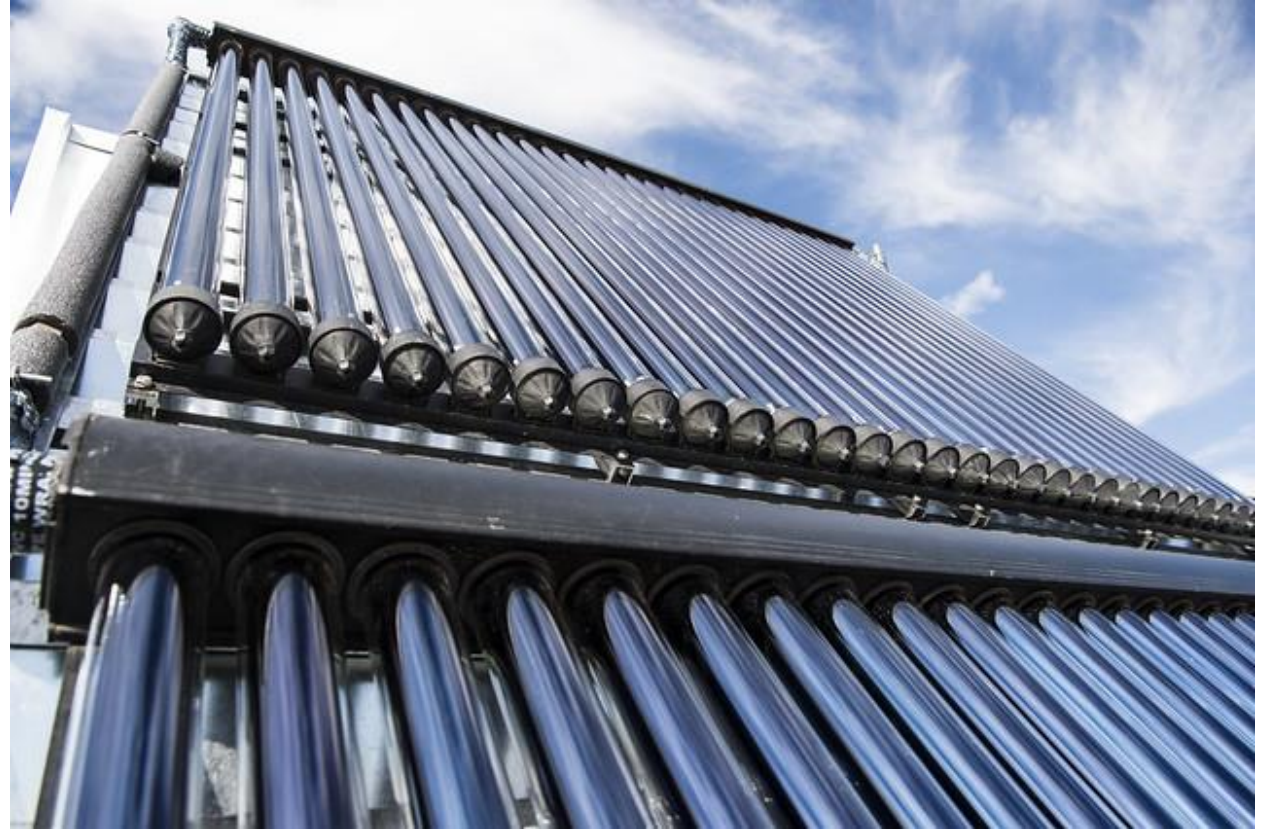
Solar thermal array. Credit: NREL .
