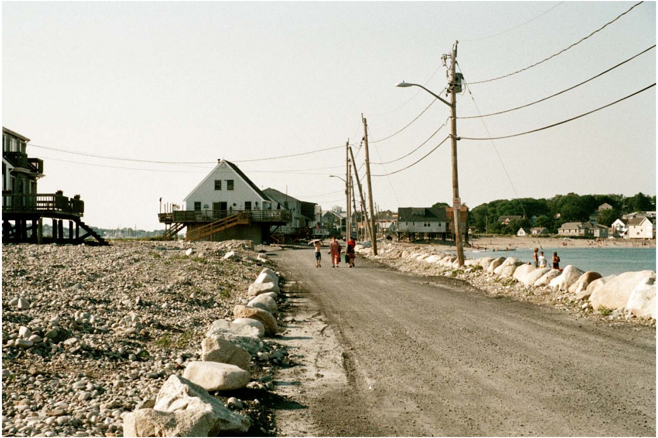
Roads, Wires, and Stone Revetment along Pegotty Beach
