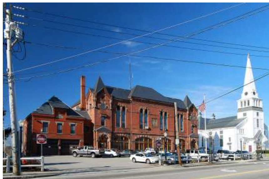
Figure 5- Powerlines over Holbrook Town Hall
