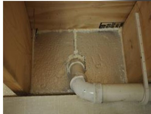
Sealing around pipes and wires blocks the flow of air
