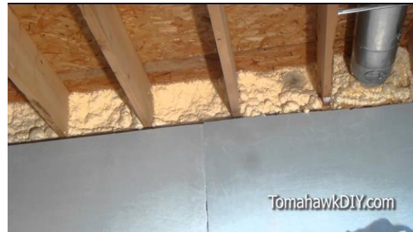
Sealing around pipes and wires blocks the flow of air
