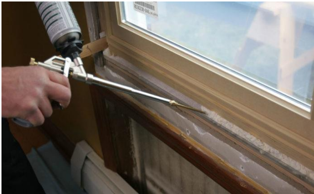
Target spray foam reduces draft around windows
