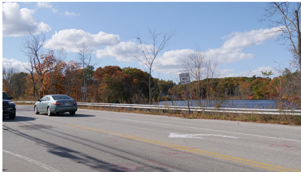
Powder Mill Road abuts the Assabet River, and a lack of stormwater controls allows drainage directly into the river
