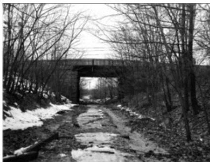
The Franklin St. Bridge over abandoned railroad, shown here from 1889, is an example of a historical engineering structure. Source: MACRIS
