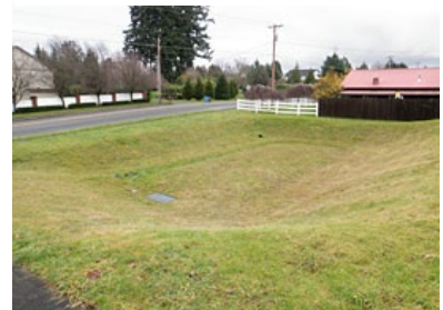
Example of a detention basin
