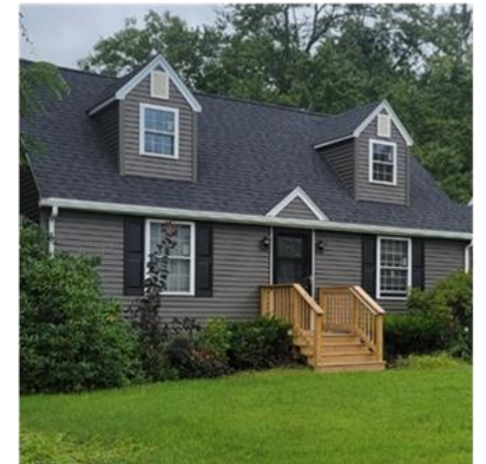
CDBG Housing Rehabilitation - after
