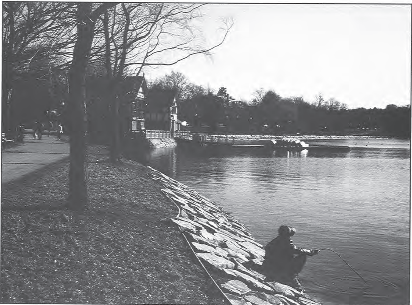
Jamaica Pond has an ongoing erosion problem, exacerbated by wave action. To stabilize the shoreline, this stone rip-rap was modeled after the original detail implemented by the Olmsted firm. (Pressley Associates and Boston Parks & Recreation)
