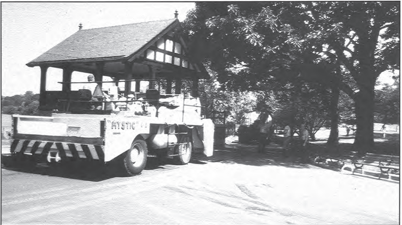
As part of a preservation project, the walks around Boston's Jamaica Pond Park were repaired and resurfaced. A loose, crushed stone surface material (an embedded aggregate) was rolled into the asphalt surface, thus allowing for upgraded uses such as jogging, biking and snow removal, while retaining the historic character. (FLONHS and author, 1990)
