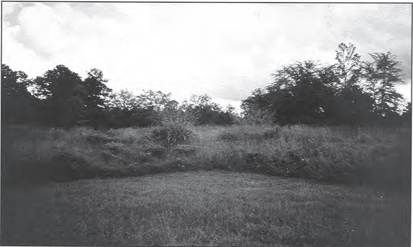
The Star-Fort at the Ninety-Six Battlefield, Ninety-Six, South Carolina, was eroding from mowing operations. [top] To remedy the situation, native grasses were installed on the historic Revolutionary War Star Fort. [bottom] The interior of the fort has been mown short to accommodate visitor access, but tall native grasses are kept longer on the earthworks to discourage visitors from walking on them and to aid in their interpretation. The difference in height of the new grasses also help to visually define the earthworks themselves. (courtesy NPS)
