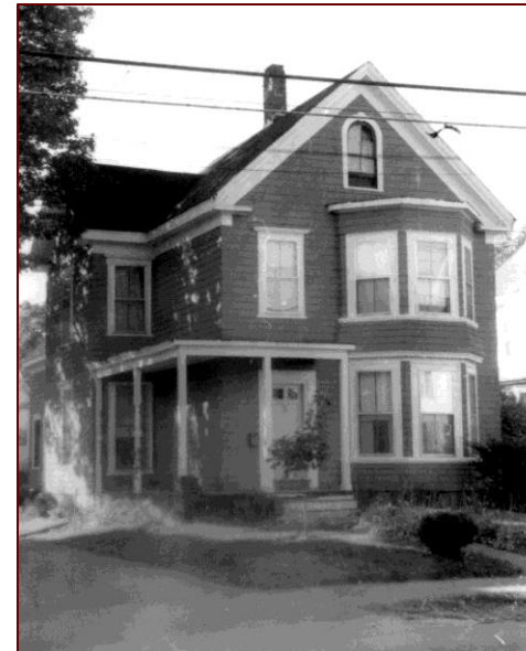
Local historic district
