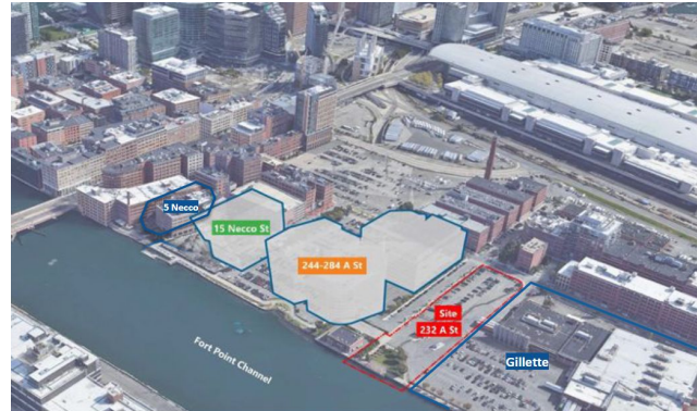
Fort Point Channel Resilience project
